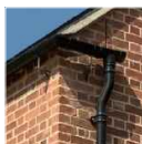
RAINWATER GOODS: Cast Aluminium
