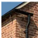
RAINWATER GOODS: Cast Aluminium
