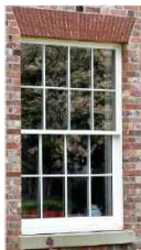
WINDOWS: Timber Sliding Sash
