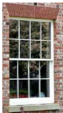
WINDOWS: Timber Sliding Sash
